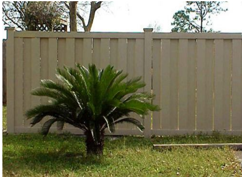
Melbourne style PVC "shadowbox" fencing.
